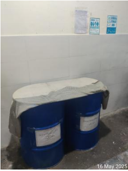
Secondary containment missing .jpg
